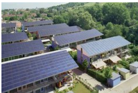
Solar PV in Freiburg, Germany, where a long-term strategy of energy conservation, CHP and renewables is benefiting the environment and the local economy
